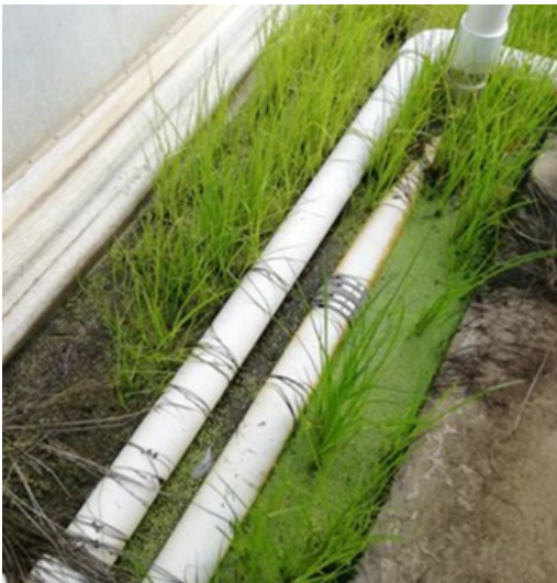
Figure 2: Exposed distribution pipes laying on wet ground.
