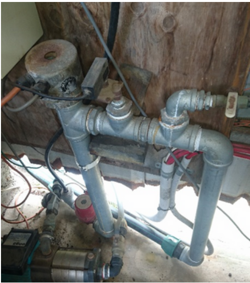
Figure 1: An un-insulated heating head
